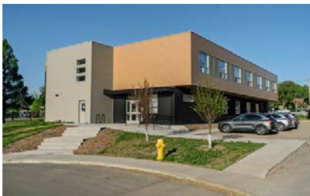
The ikwēskīkik iskwēwak transitional housing facility in Saskatoon.
