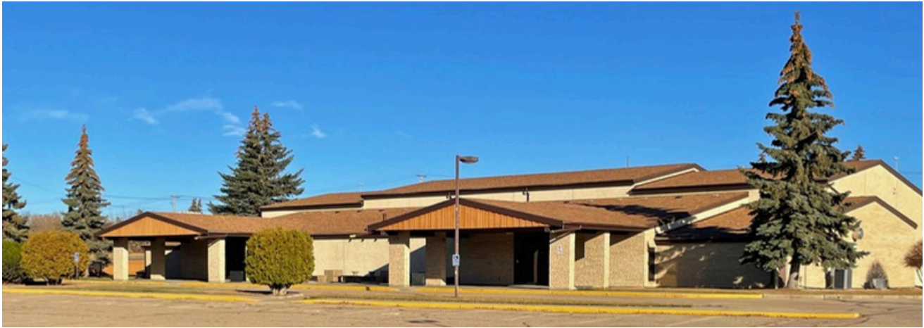
The Saskatoon Tribal Council's Emergency Wellness Centre offers 106 emergency shelter beds and access to STC programs and supports, along with programs and services offered by government and community partners.
